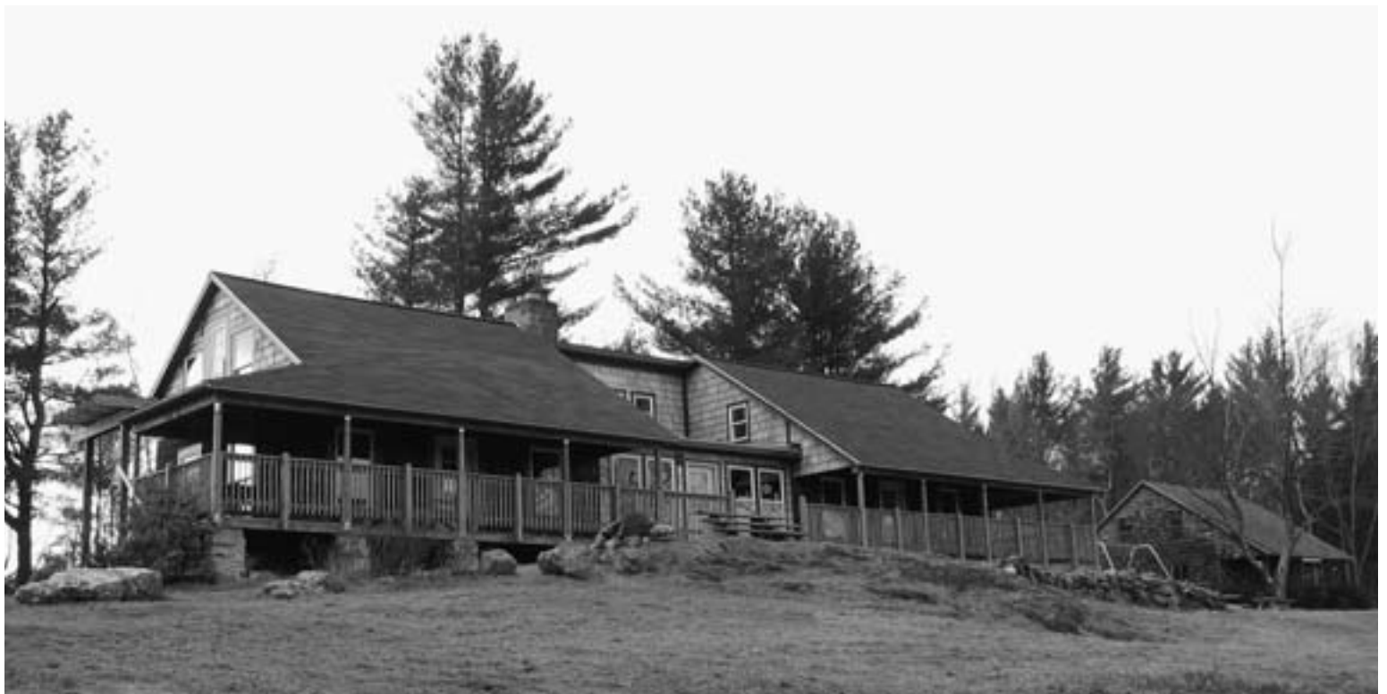
Noble View Camp's Double Cottage and North Cottage. photo by Jon Hanauer
